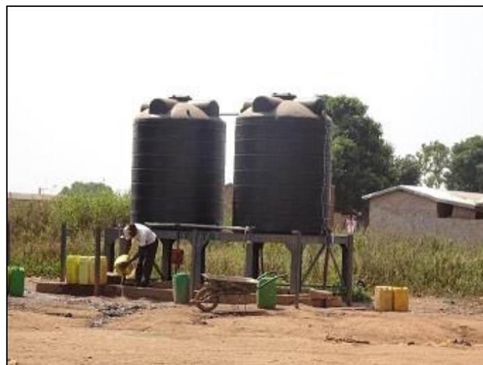
Figure 20-3 Water Tanks at Fadiadougou
